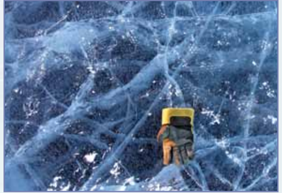
Cracks in the TCWR ice road found during an inspection
