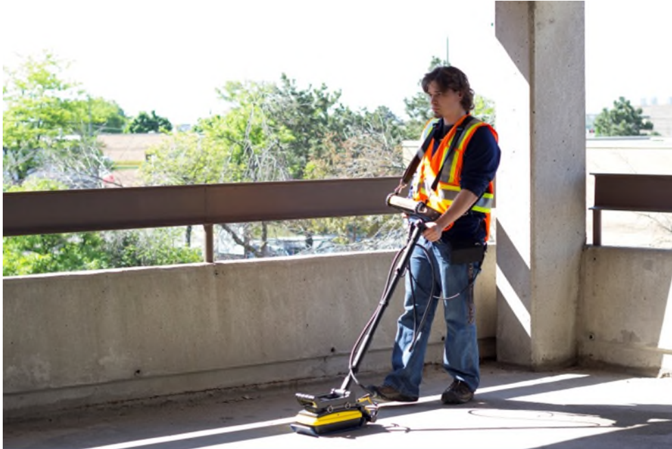
Figure 2-64: SmartHandle with harness on a site
