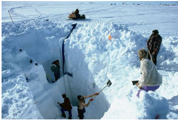
Hand excavation of snow at the surface to establish the start of the excavation shaft.
