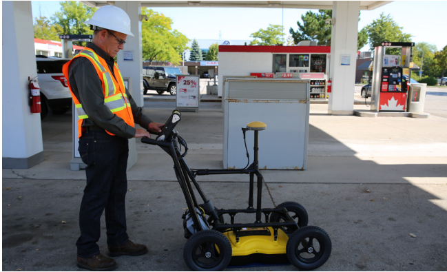
Surveying the gas station with the Noggin 250 SmartCart.
